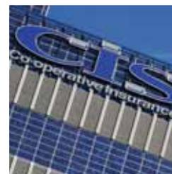
**The Co-operative Solar Tower, Manchester.** The Co-operative Insurance head office is clad in 7,000 photovoltaic cell panels, which have the potential to save 78 tonnes of CO<sub>2</sub> emissions each year.
